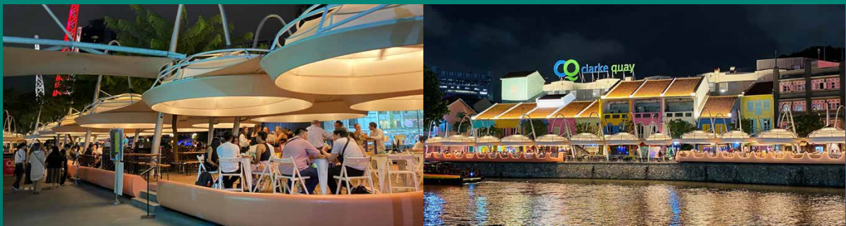
Completed upgrading of the outdoor refreshment area along Singapore River
